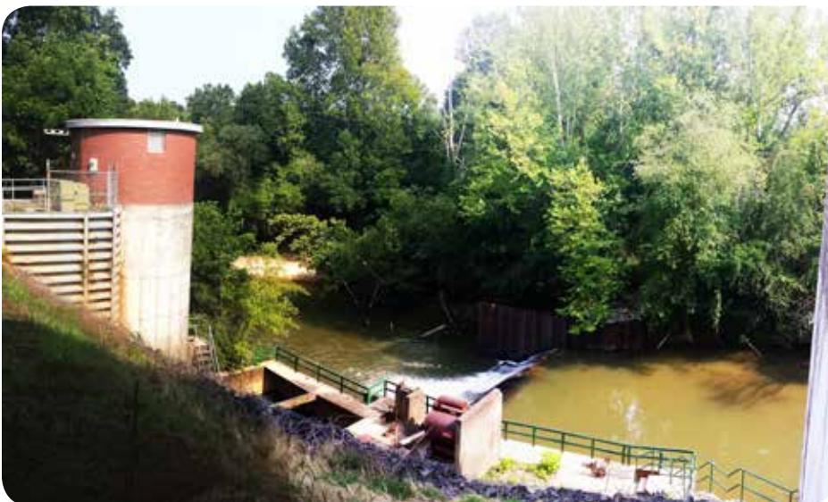
FIGURE 3.21: Examples of utility services located within the Polkville Road Interchange study area: Wal-Mart Distribution Center Lift Station and the City of Shelby Water Intake .
