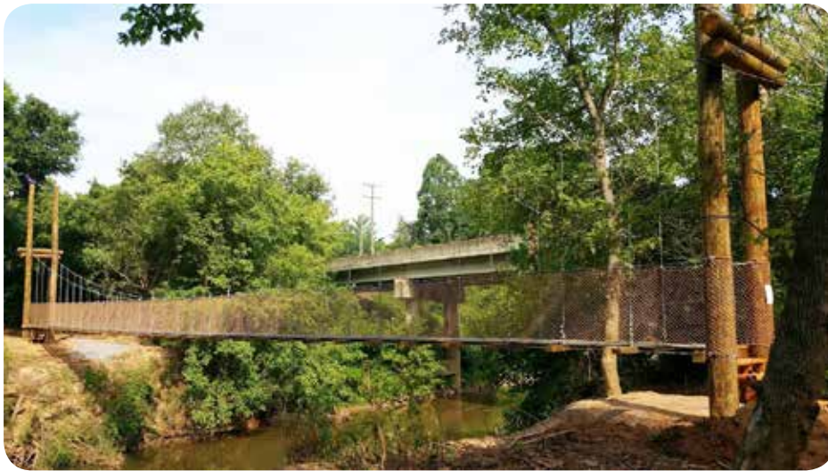
FIGURE 5.5.: Pedestrian bridge under construction for the Carolina Thread Trail that crosses the First Broad River and a portion of the trail. With the completion of this bridge, there is an opportunity to expand the Carolina Thread Trail west of Shelby through the Polkville Road Interchange study area.
