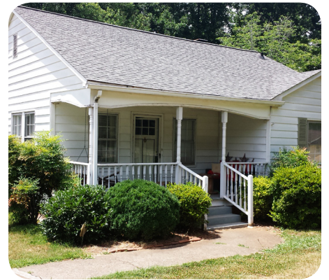
Residential along Polkville Road.
