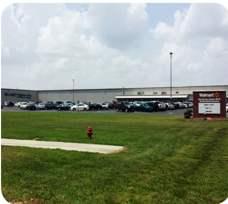
The Wal-Mart Distribution Center off of Polkville Road.
