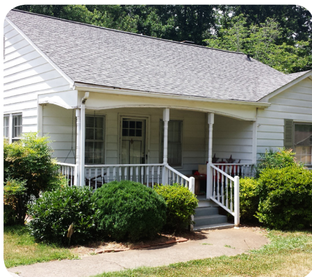
A residential property along Polkville Road.
