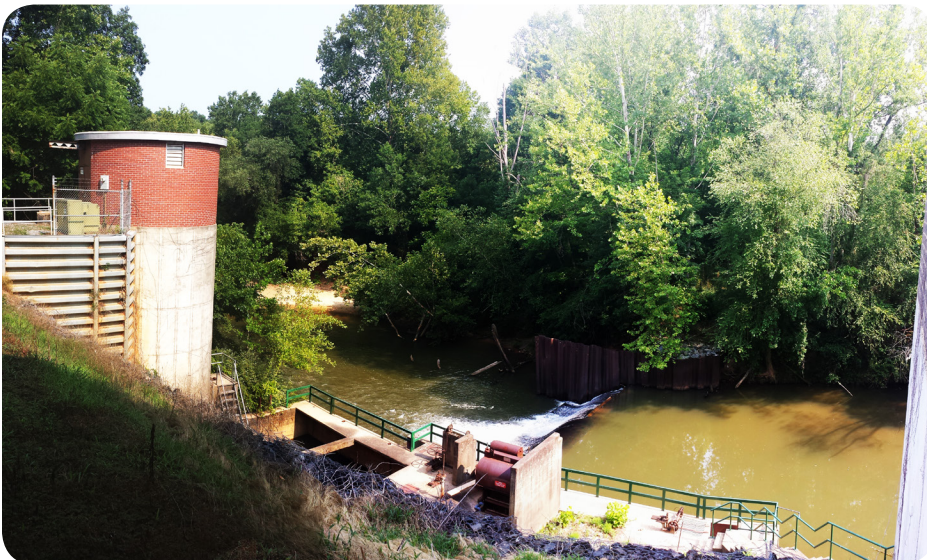
FIGURE 3.21: Examples of utility services located within the Polkville Road Interchange study area: Wal-Mart Distribution Center Lift Station and the City of Shelby Water Intake .
