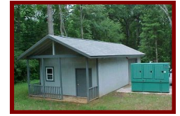
Sewer Lift Station
