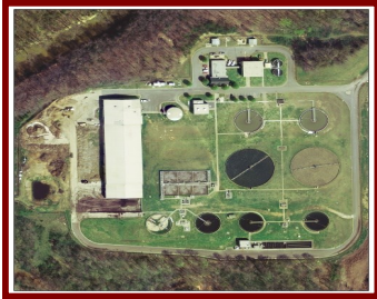
Aerial View of the First Broad River WWTP
