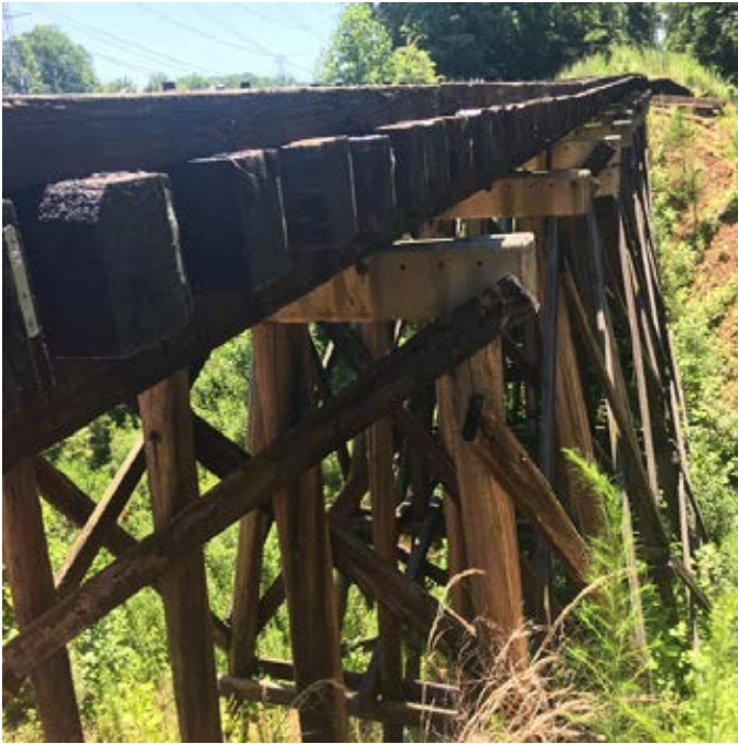
Second rail trestle bridge.
