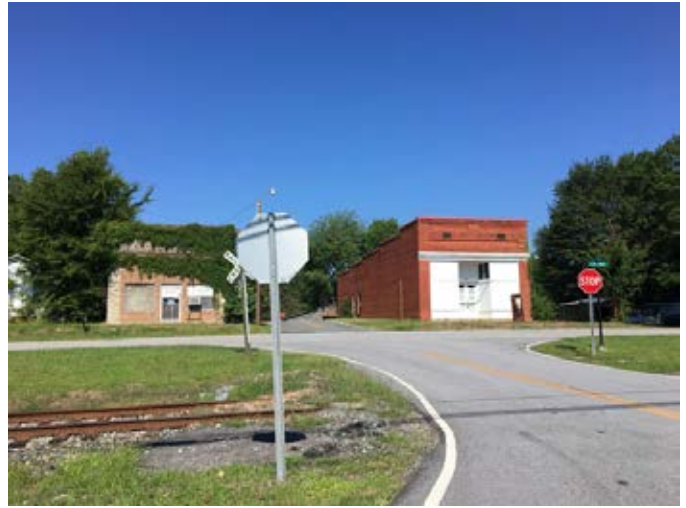
Commercial buildings in Earl
