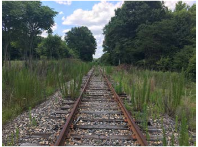
Existing conditions at typical rail trail section.
