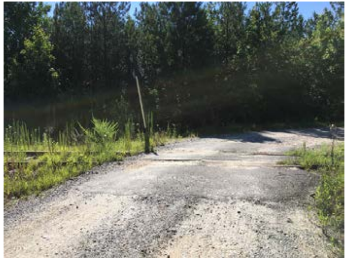
Existing conditions at Ross Road crossing.
