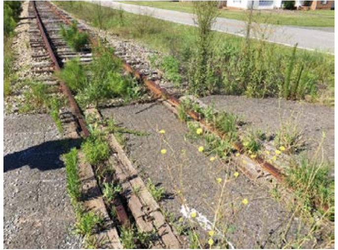
Existing conditions at driveway crossing.
