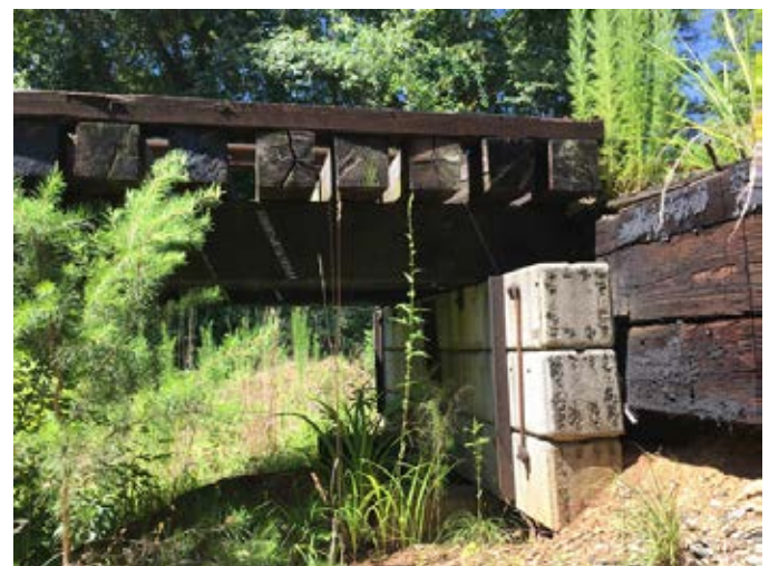
First rail trestle bridge.
