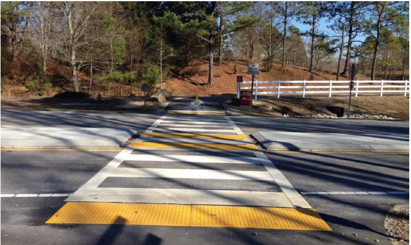
An example of an at-grade roadway intersection
