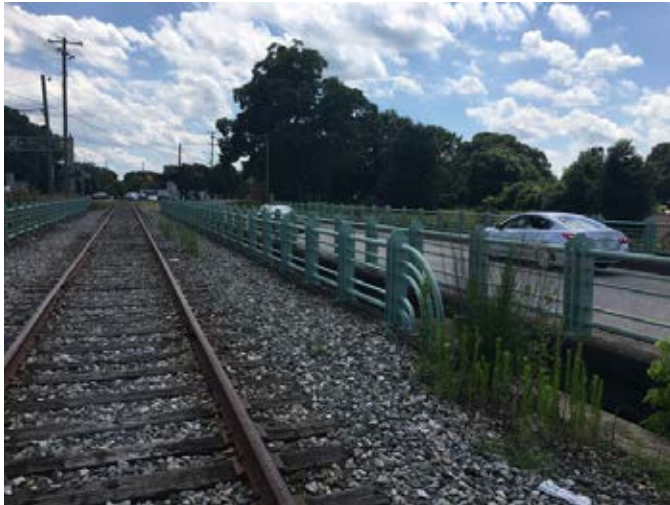
Railroad bridge over US 74.
