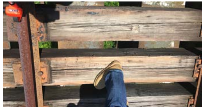
Rail, trestle and girders at third rail trestle bridge.
