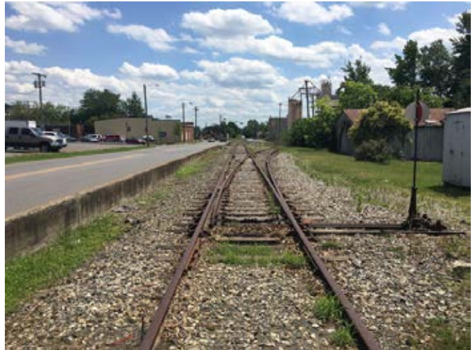
Corridor parallel to South Morgan Street near Historic Depot.
