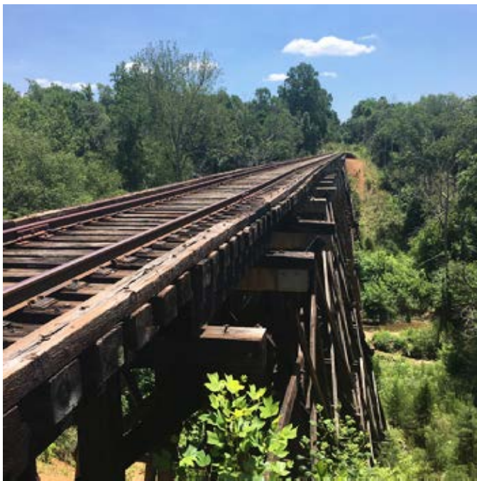
Third rail trestle bridge.
