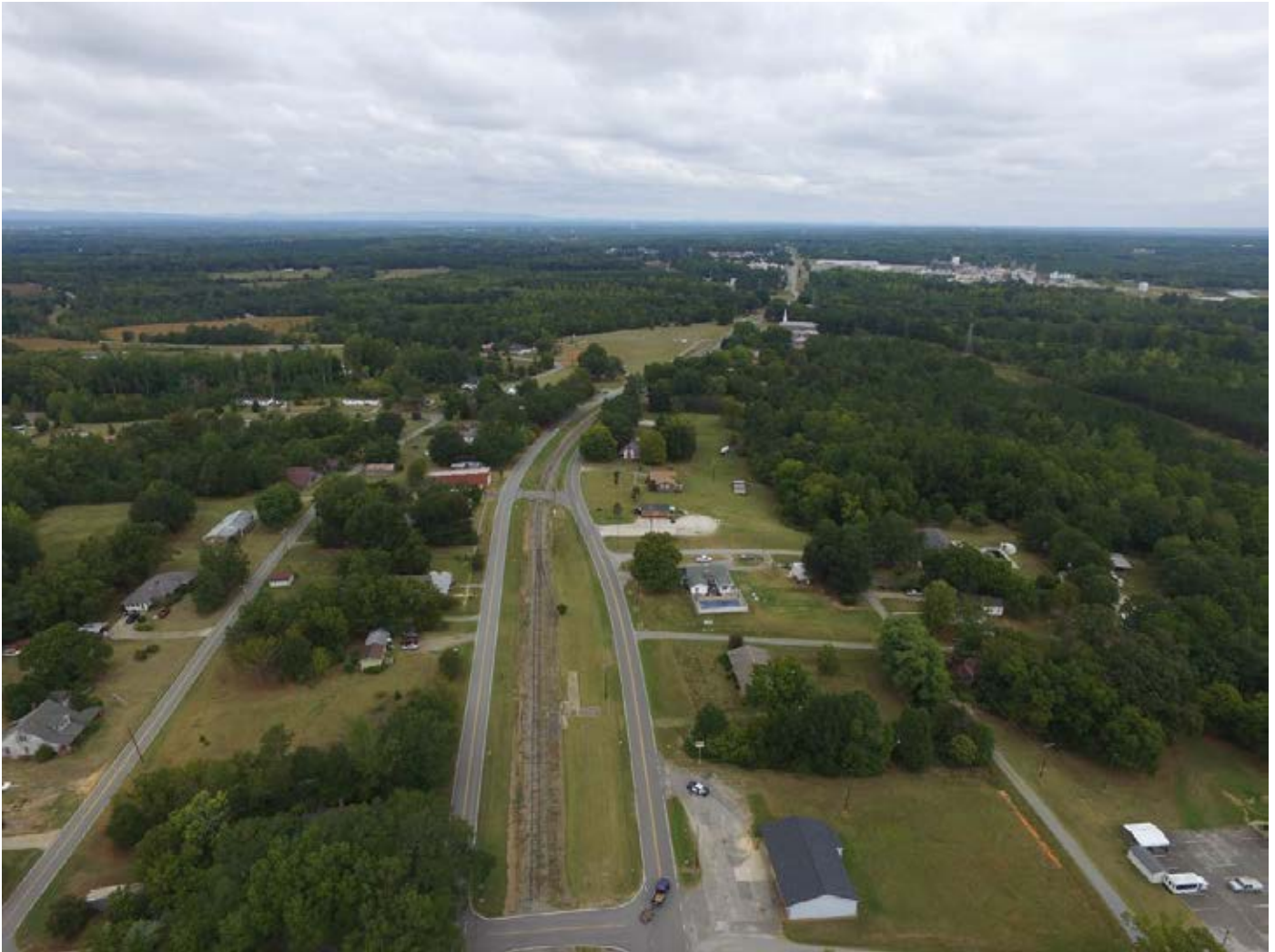
Existing conditions in Earl.
