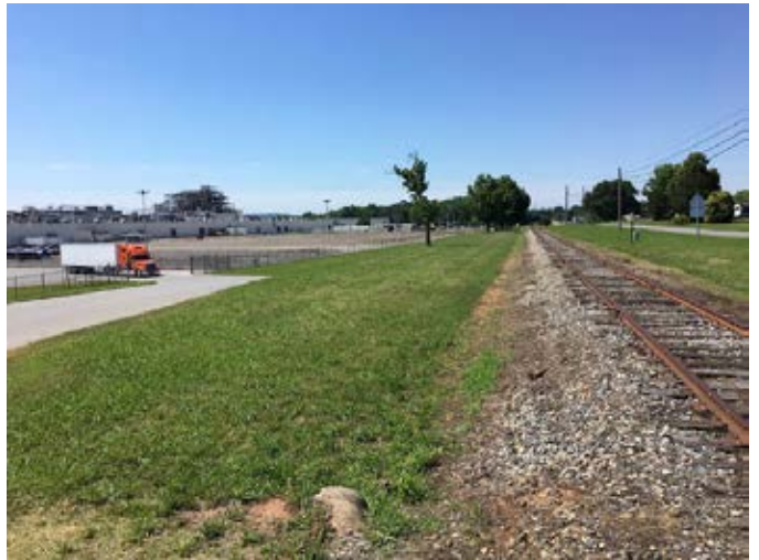
Existing conditions at Celanese.
