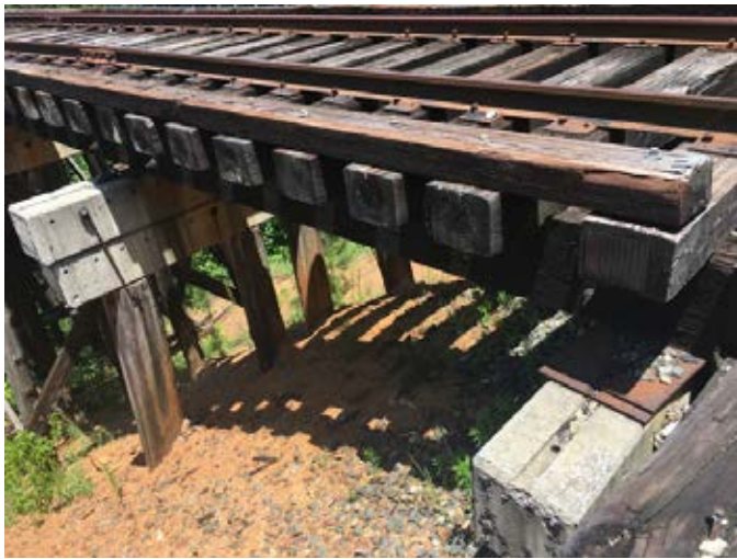
Steel shims at third rail trestle bridge.
