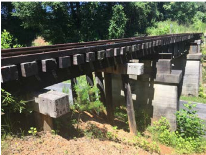
First rail trestle bridge.
