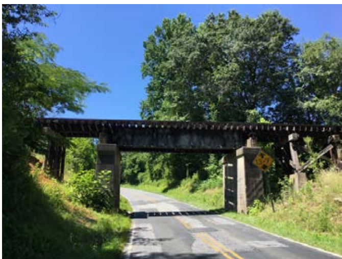
First rail trestle bridge.
