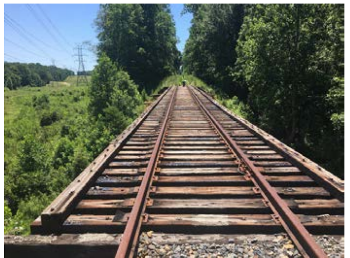
Second rail trestle bridge.
