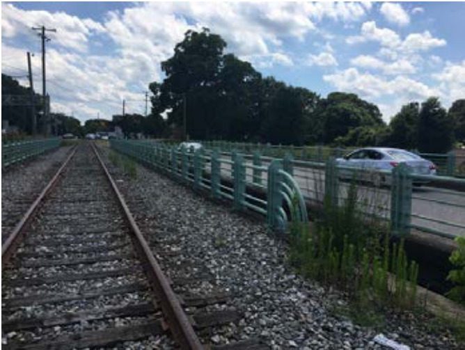
Railroad bridge over US 74.
