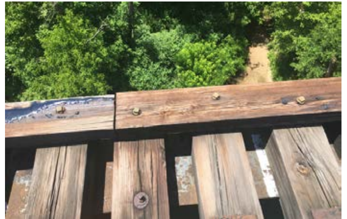
Edge of third rail trestle bridge.
