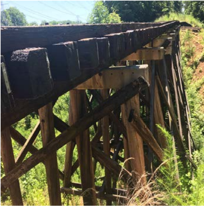
Second rail trestle bridge.
