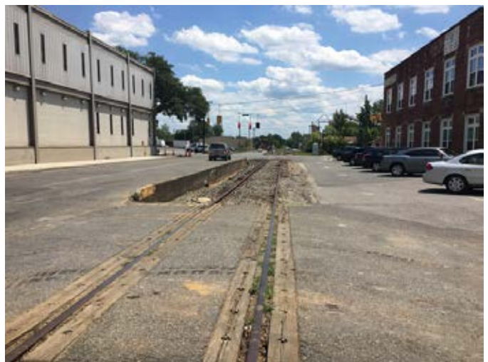
Corridor parallel to S Morgan Street at City Farmers Market building.
