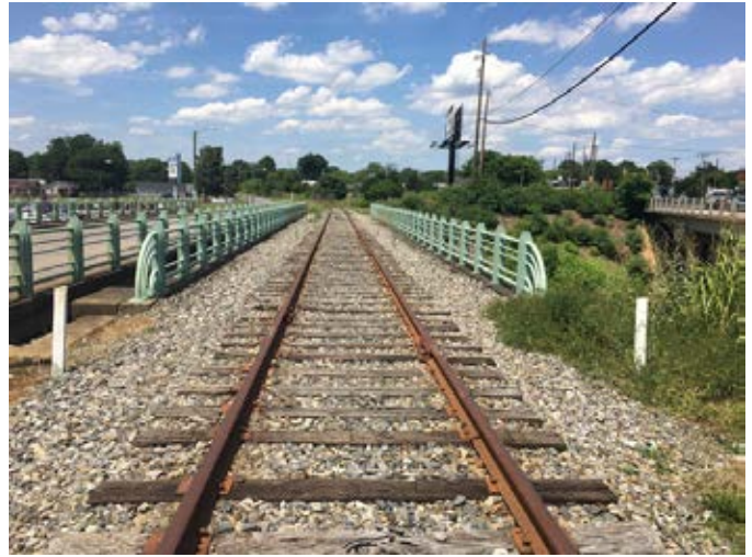
Existing conditions at bridge over US 74.
