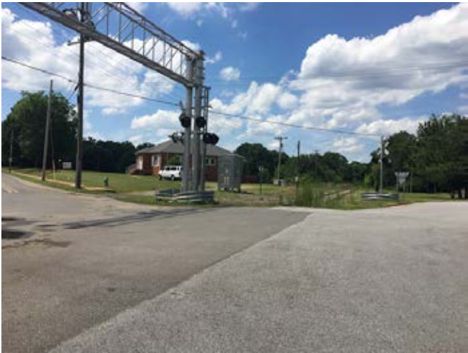
Morton Street crossing.
