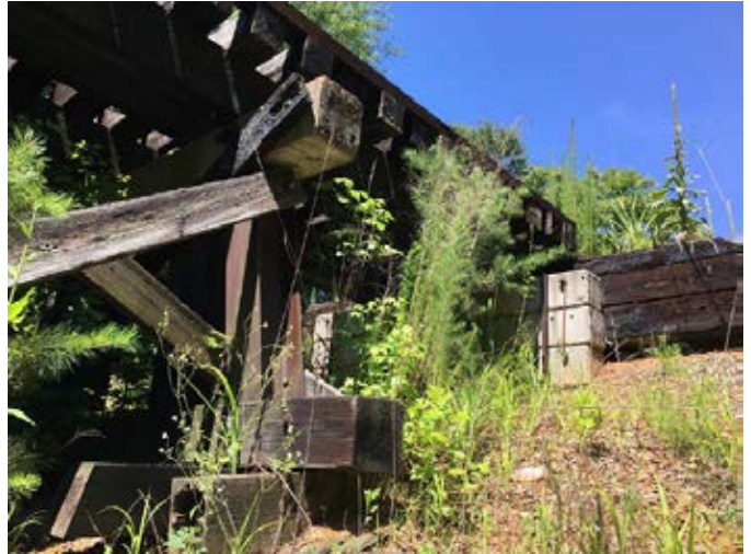
Existing conditions at rail trestle bridge 1.
