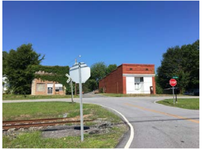
Commercial buildings in Earl
