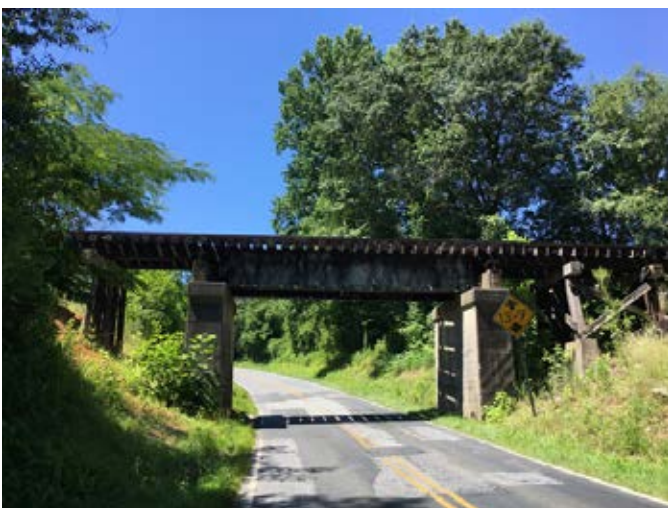
First rail trestle bridge.
