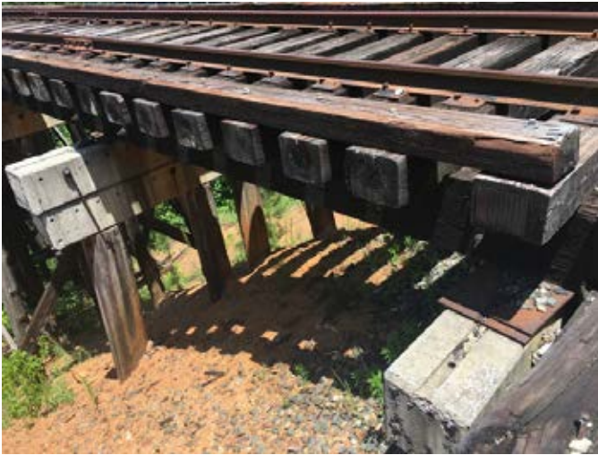
Steel shims at third rail trestle bridge.
