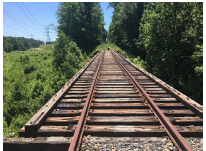
Second rail trestle bridge.
