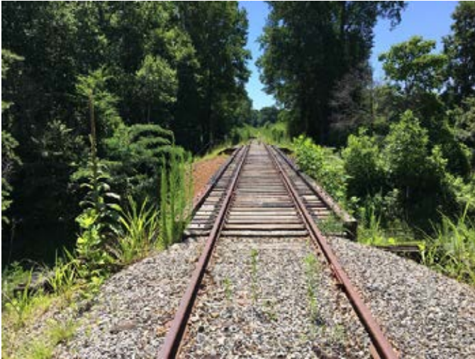
Existing conditions at rail trestle bridge 1.
