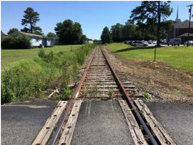
Existing conditions at Ellis Chapel Baptist Church.
