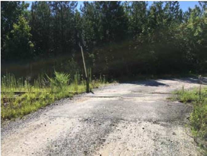
Existing conditions at Ross Road crossing.
