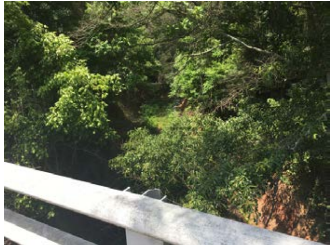
W Sumter Street bridge over rail corridor.
