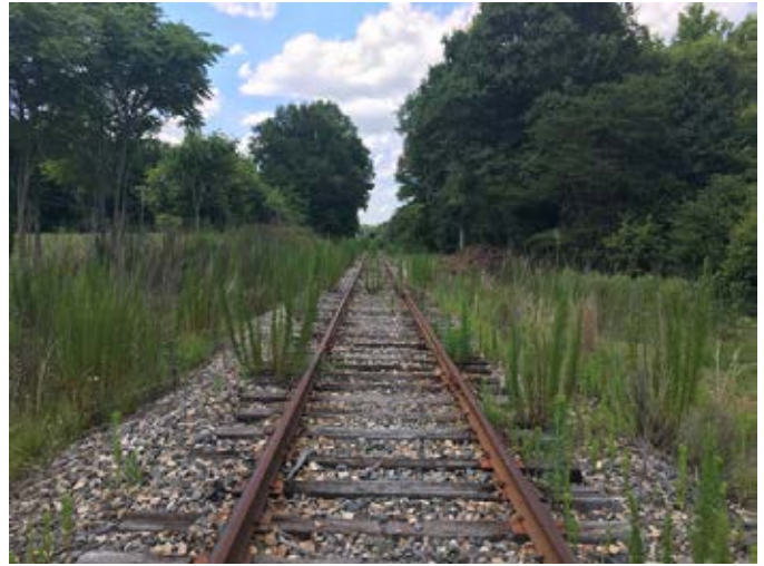
Existing conditions at typical rail trail section.
