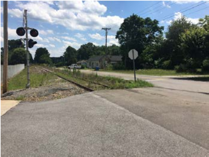
Morton Street crossing.
