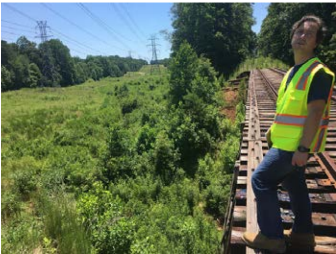
Existing conditions at rail trestle bridge 2.
