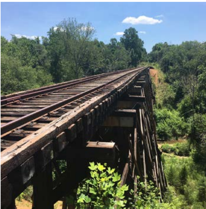
Third rail trestle bridge.
