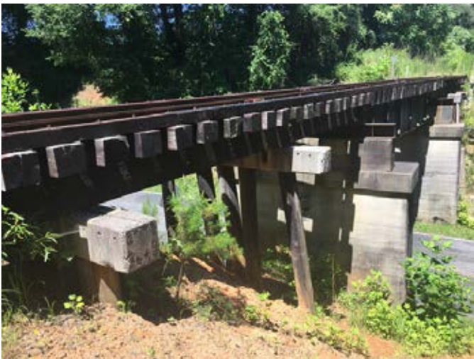
First rail trestle bridge.
