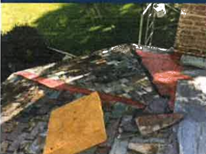
START OF REPAIRS
