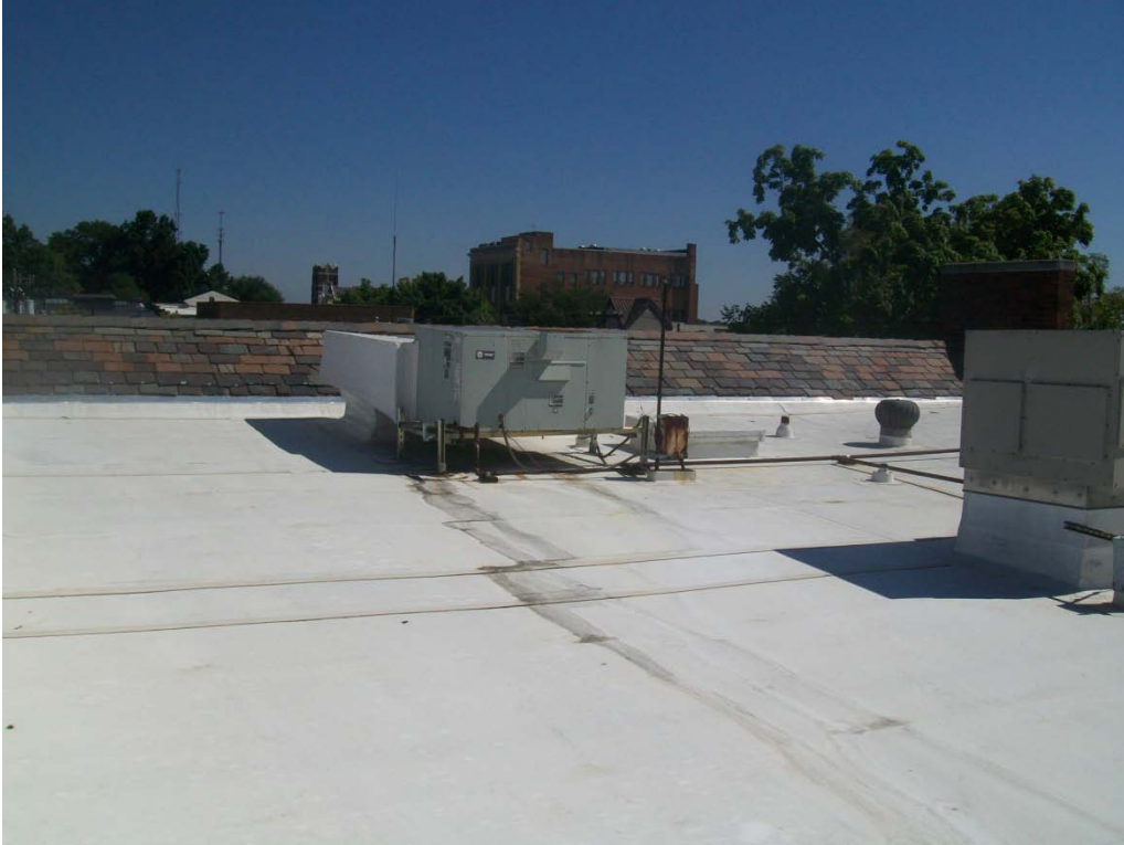
Photo 29: Area J Overview
