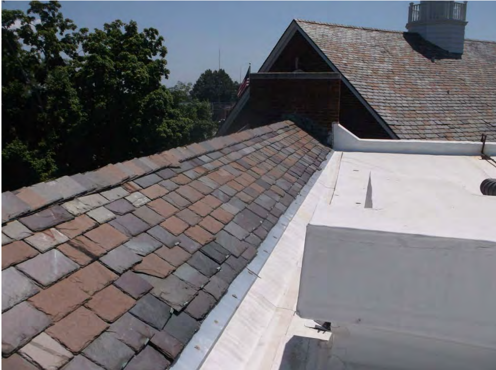
Photo 30: Transition from Area I to Area J
