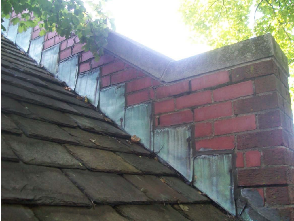
Photo 13: Typical Step Flashing and Counter Flashing Condition
