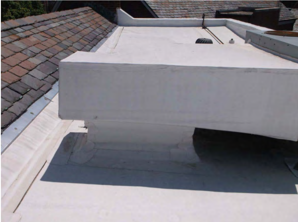
Photo 28: Area J Overview
