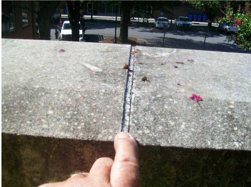
Photo 32: Typical Cast Stone Coping Joint
