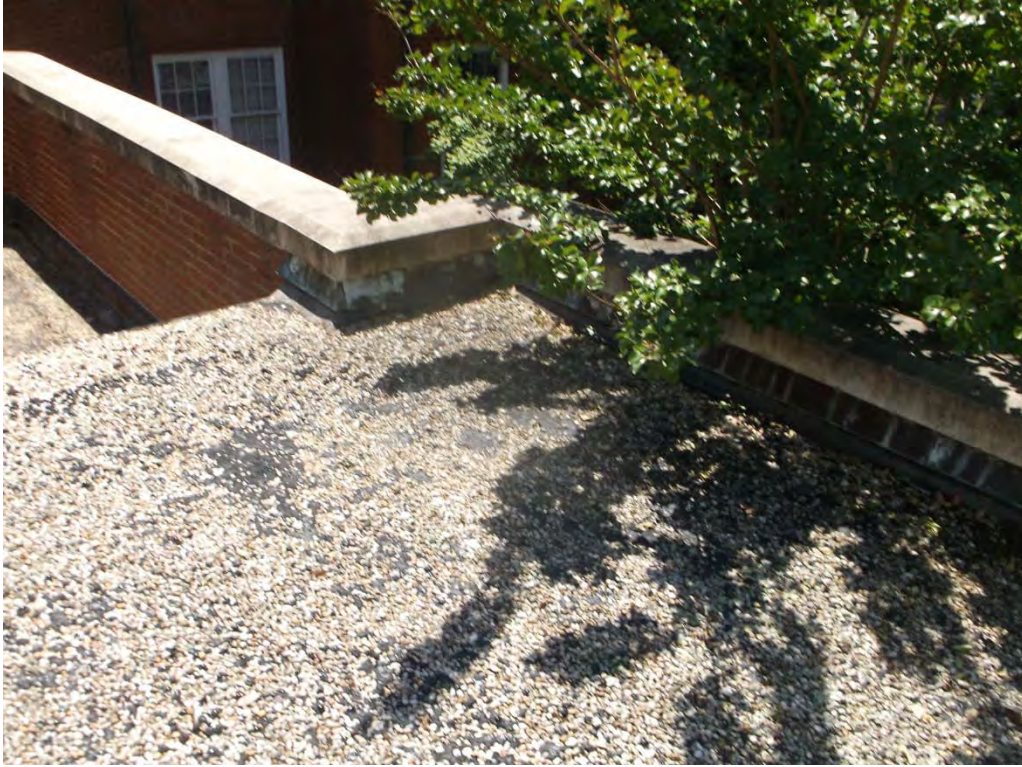
Photo 31: Typical Cast Stone Coping
