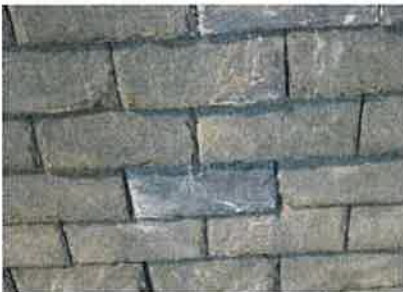
SHOWING REPAIRED SLATE
