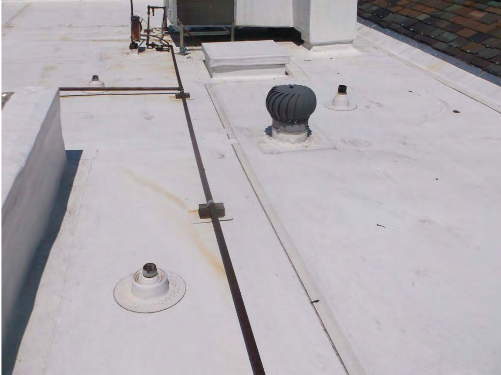
Photo 27: Area J Overview
