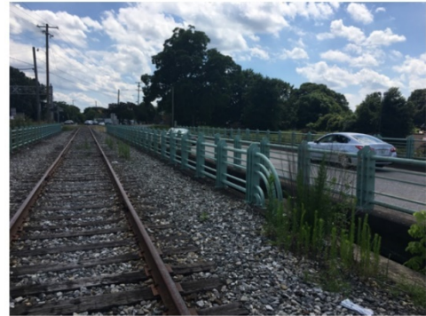
Railroad bridge over US 74.
