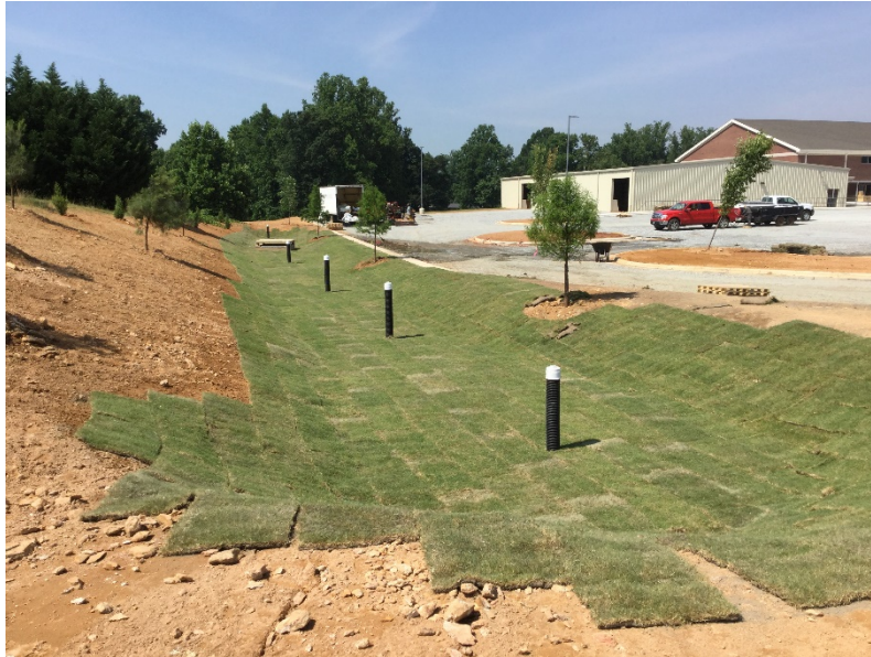
Bioretention cell under construction at a local school
