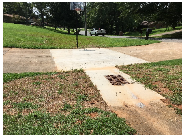
Poplar Circle Project After Repairs
