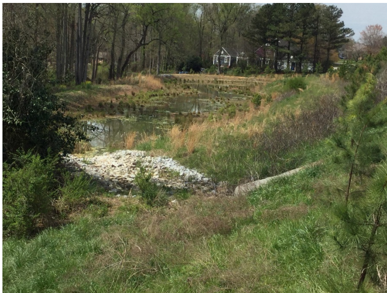
Constructed wetland at the Cleveland County Health Department
