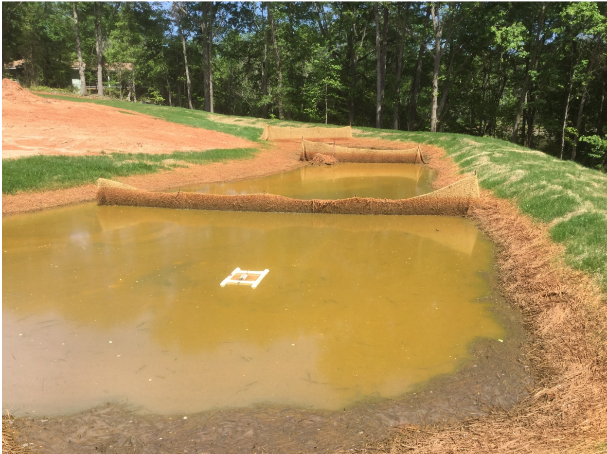
Sediment basin at a local construction site
