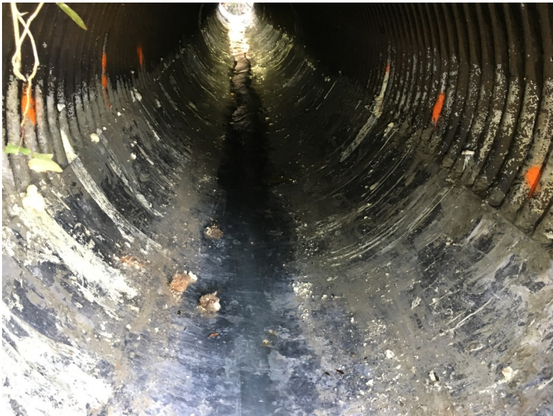
Westover Terrace Culvert- after plating
