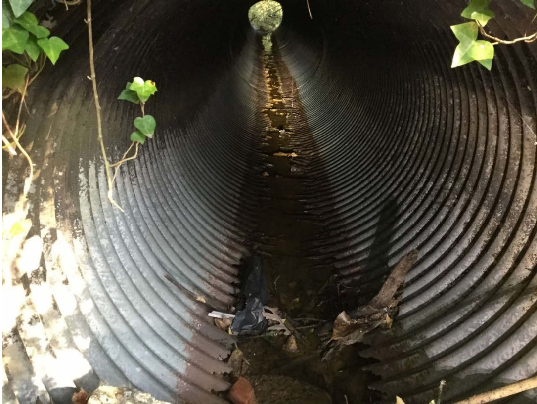
Westover Terrace Culvert- before plating
